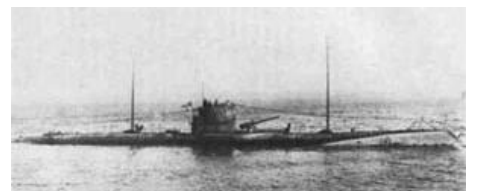
U-Boat Speed: 13 knots surfaced/ 7.4 submerged Seats: 25 Diving Depth: 250 feet Range: 1600 Miles
